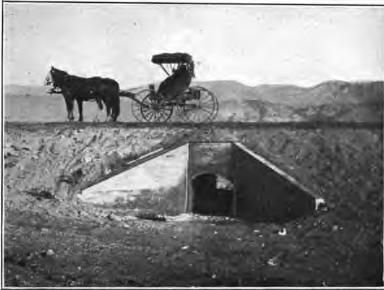
CONCRETE CULVERT, STATE ROAD, PIUTE COUNTY.
